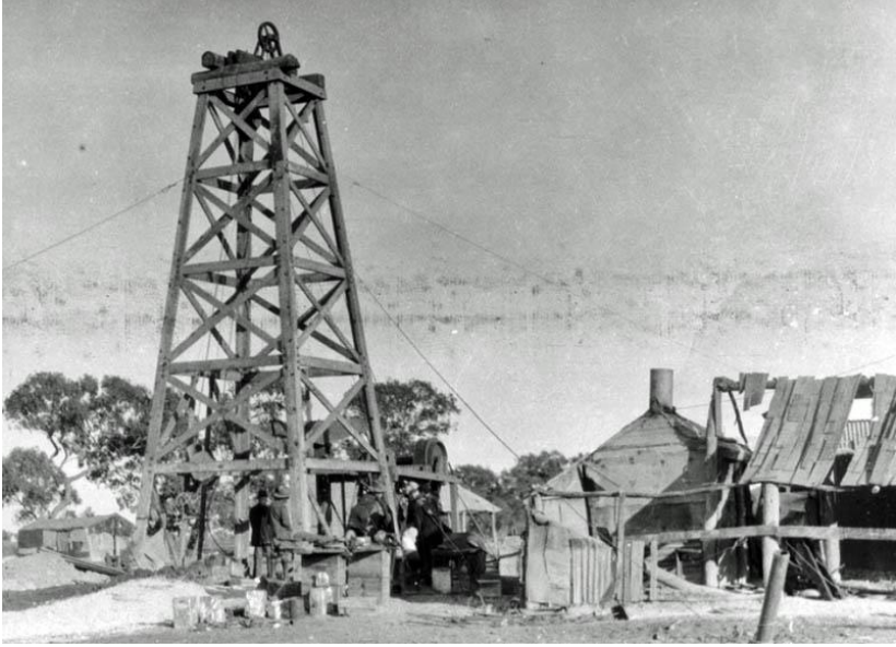
Bore sinking, 1921. (State Library of SA, PRG 1365/1/460)
