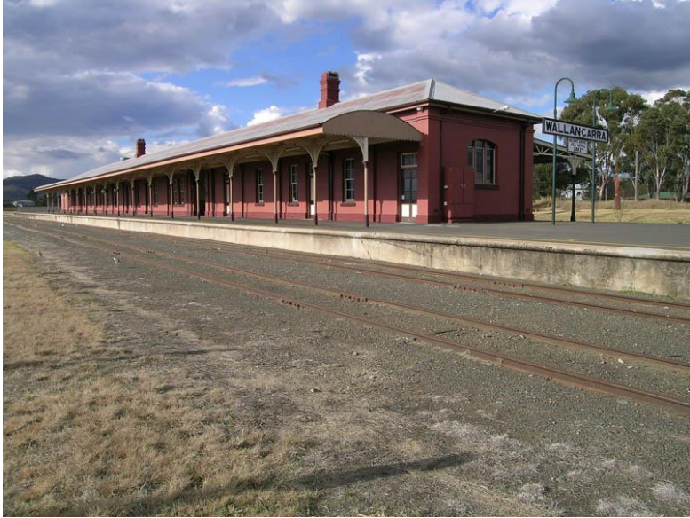
Wallangarra Railway Station. By Cgoodwin - Own work, CC BY-SA 3.0, https://commons.wikimedia.org/w/index.php?curid=4175069
