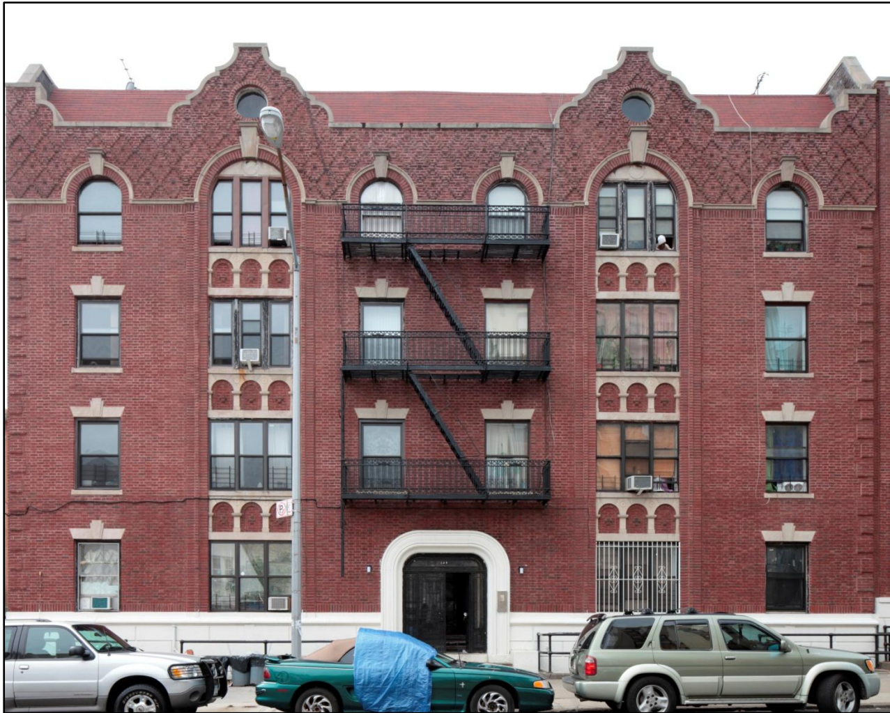
Figure 30 940 Prospect Place John C. Wandell Company, 1916-17 Photo: Christopher D. Braze, 2011
