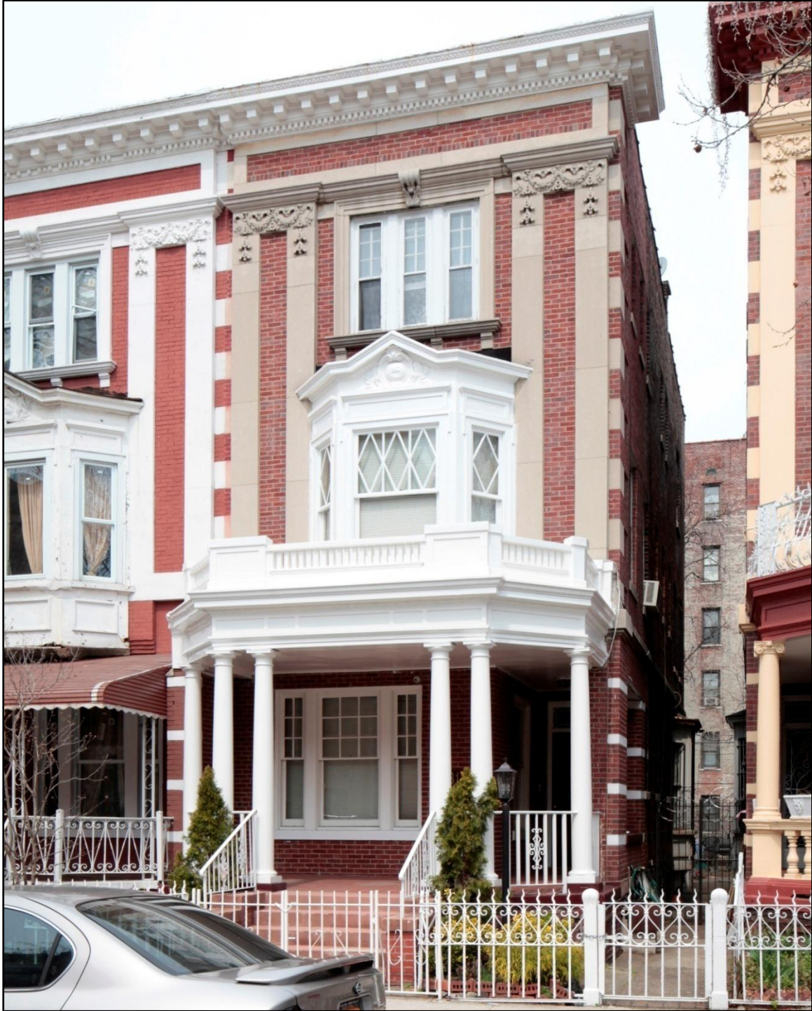
Figure 23 817 Prospect Place Attributed to Axel S. Hedman, c. 1907 Photo: Christopher D. Brazee, 2011
