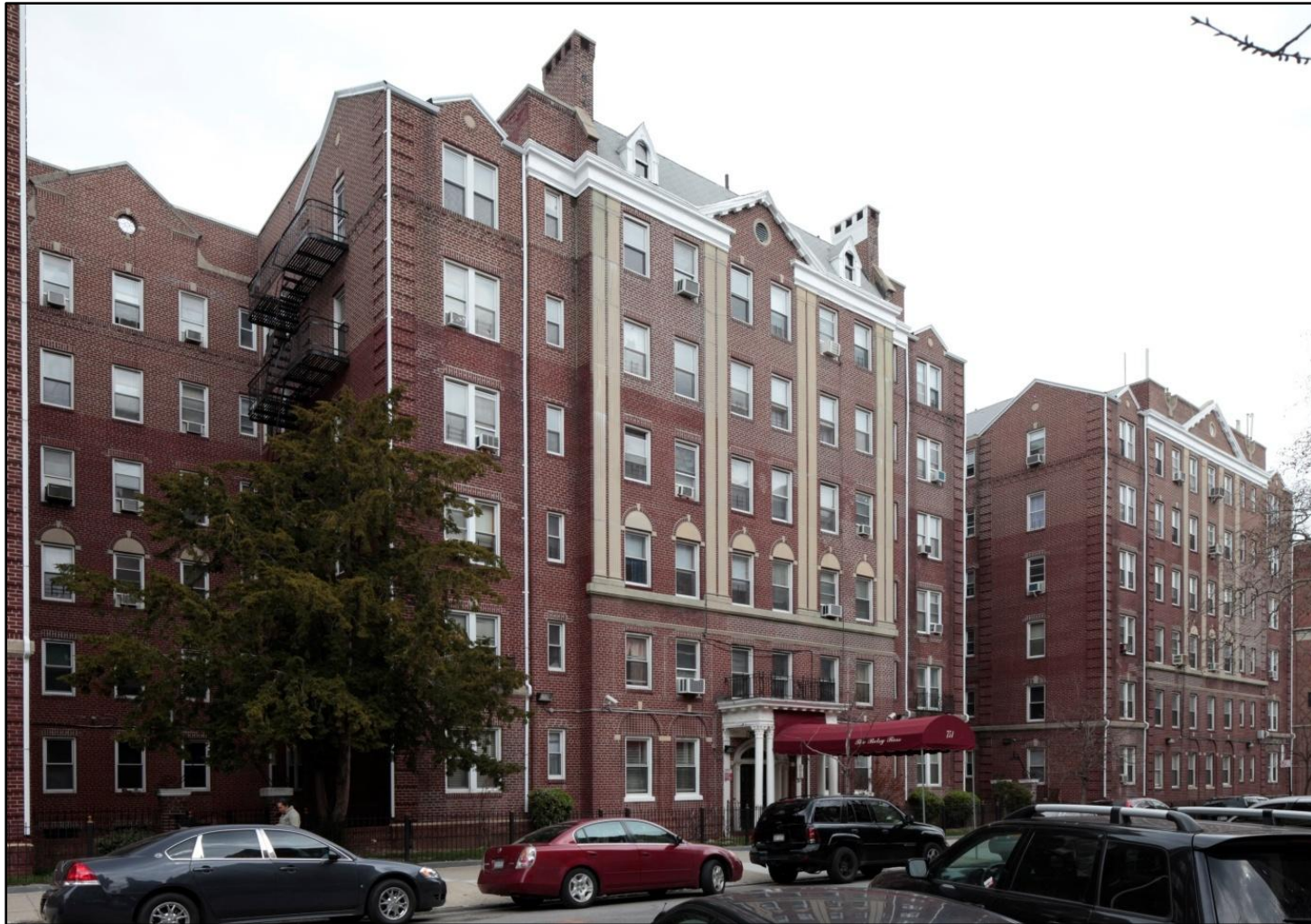
Figure 46 Betsy Ross Apartments, 751 St. Mark's Avenue Cohn Brothers, 1935-37 Photo: Christopher D. Brazee, 2011
