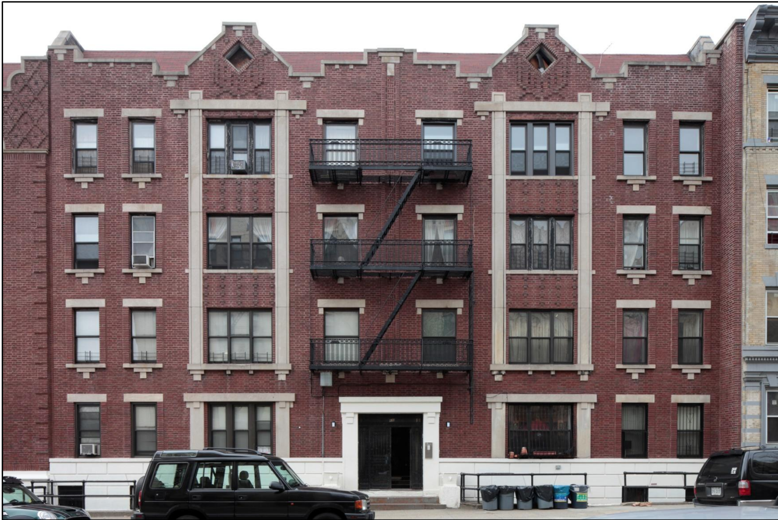
Figure 29 930 Prospect Place John C. Wandell Company, 1916-17 Photo: Christopher D. Braze, 2011
