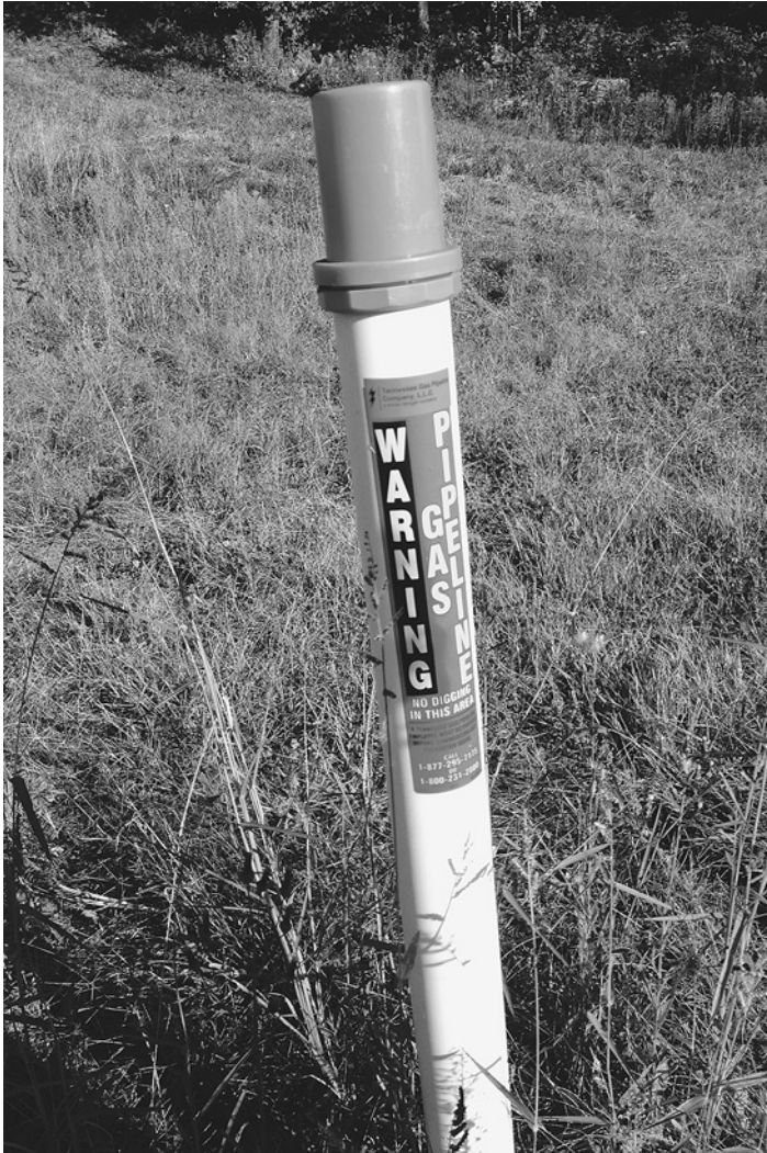
Figure 2.16. Gas pipeline infrastructure encountered during walk with participants. Photograph by Citizen Sense.
