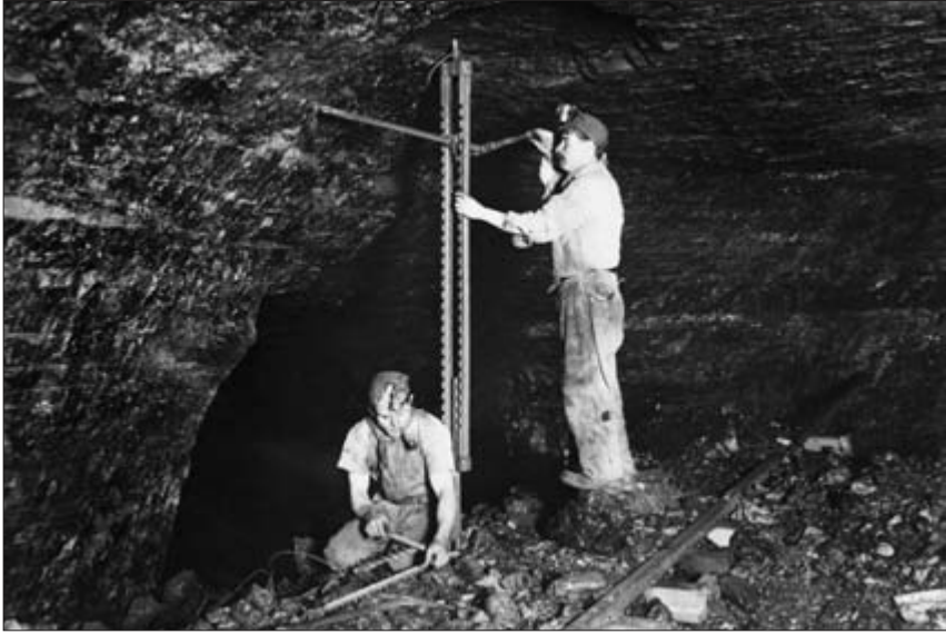
Castle Gate miners handdrilling to set dynamite, 1920
