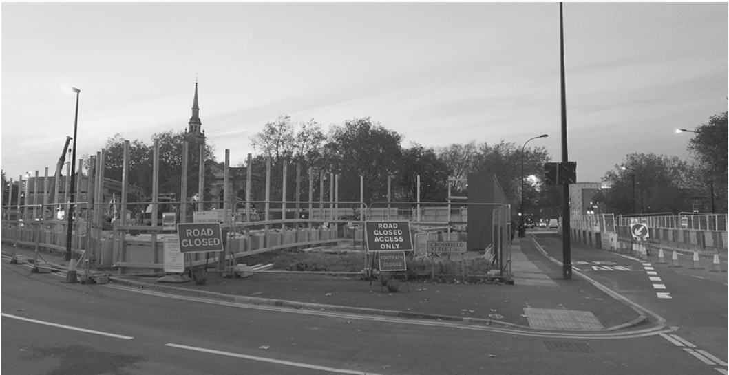
Figure 3.16. Thames Tideway Super Sewer construction. Photograph by Citizen Sense.
