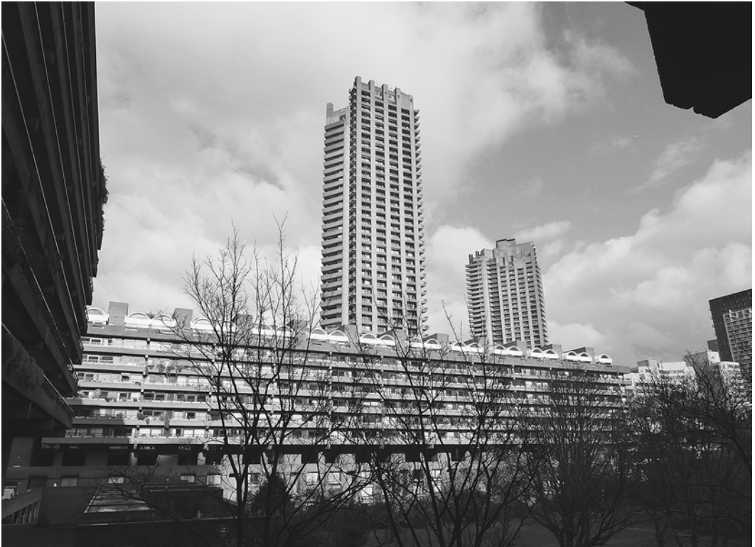
Figure 4.5. Construction on the perimeter of the Barbican; internal gardens at the Barbican in the City of London. Photographs by Citizen Sense.
