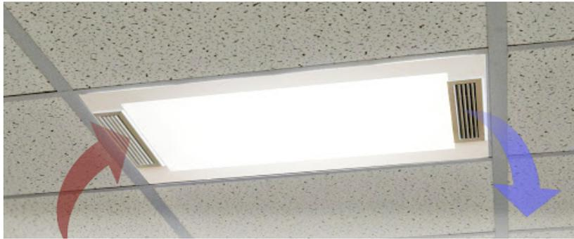
Fig. 14. Ceiling-mounted UV-C air purifier [28].
